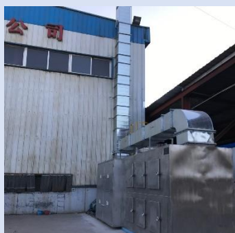
Shanxi Tube-Cote set up VOCs treatment devices which address more than 95% of waste gases.
